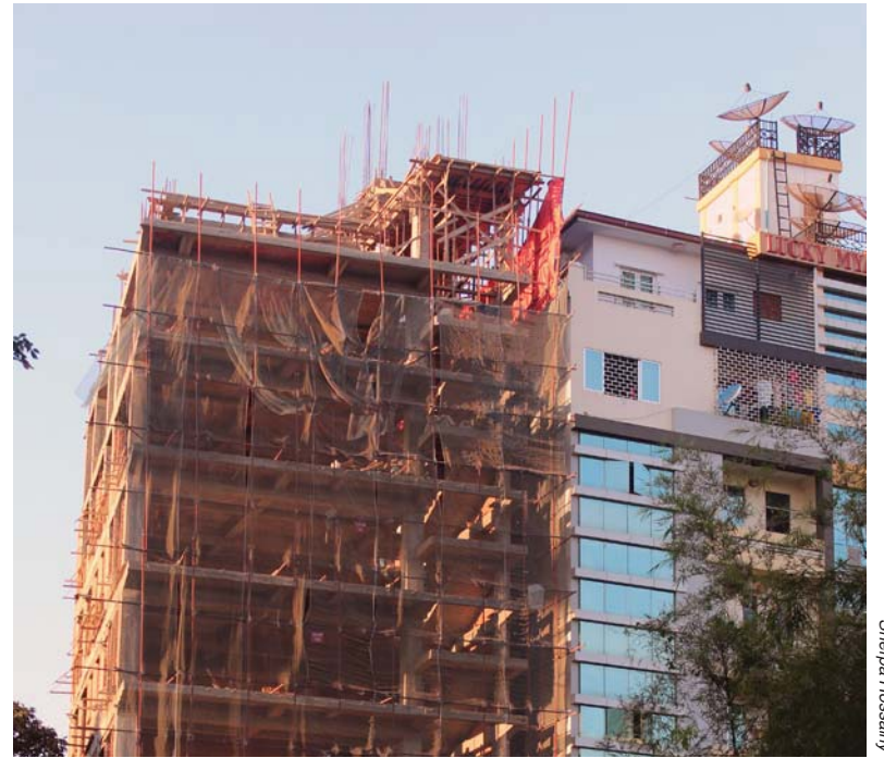
A building under construction in Yangon.
