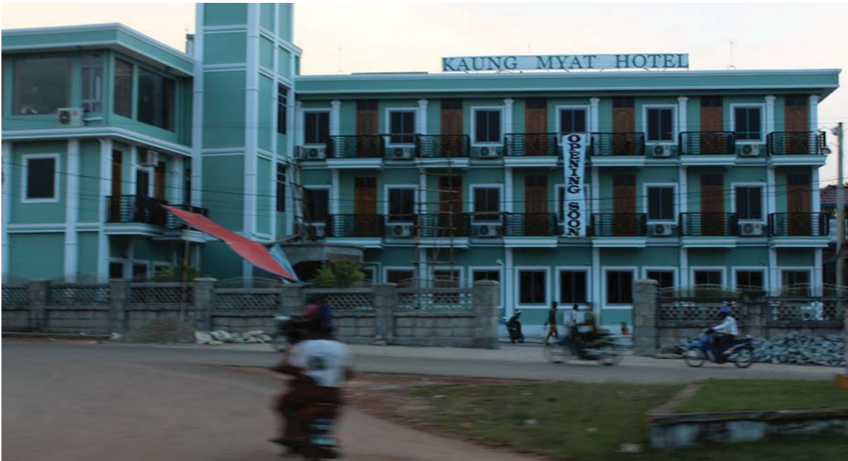
An under-construction hotel in Mawlamyine, Mon state, Myanmar.
