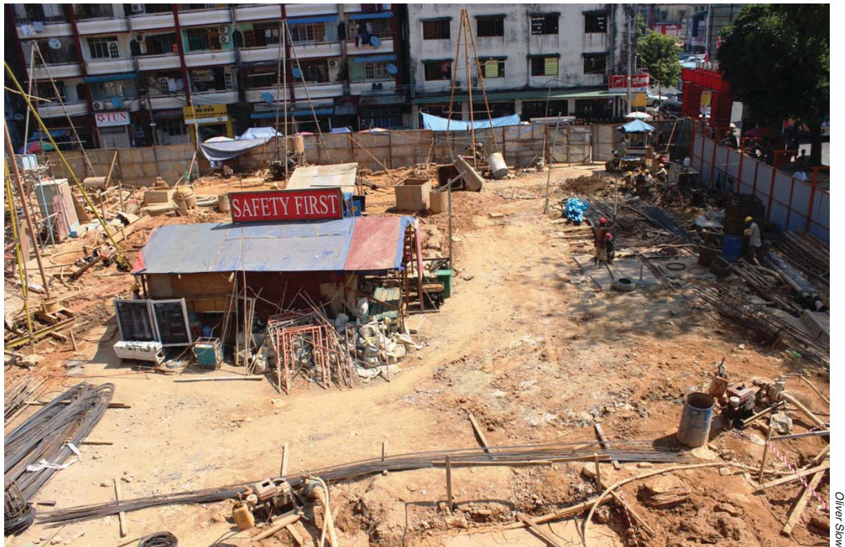
A hotel construction site in Yangon.
