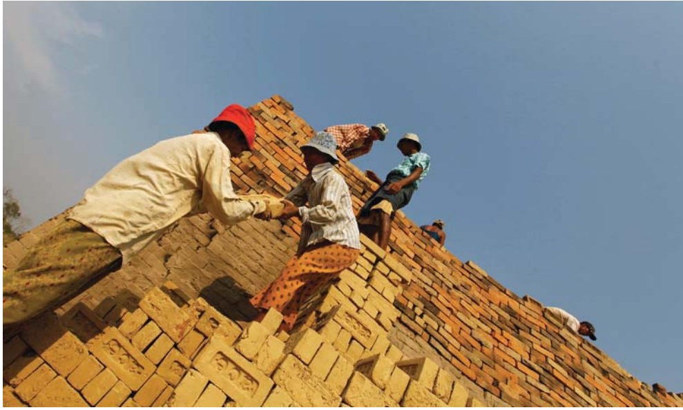
Labourers work at a construction site in Myanmar.
