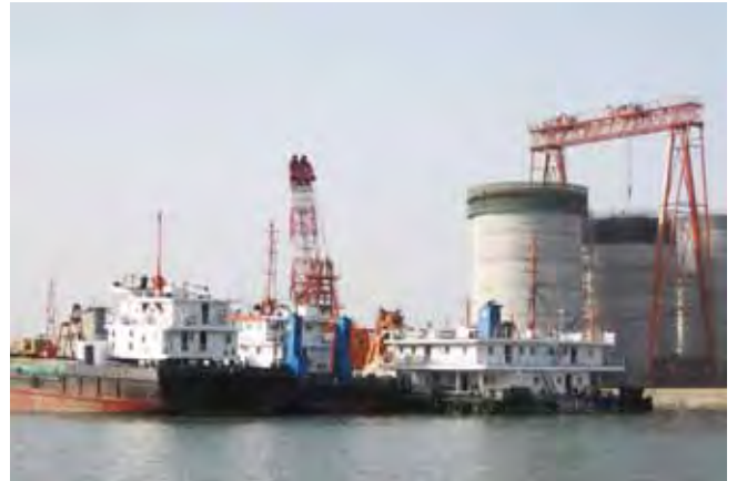
Construction of China's seaport at Madaay Island, Kyauk Phyu Township.
